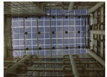
View of PV roof from below
